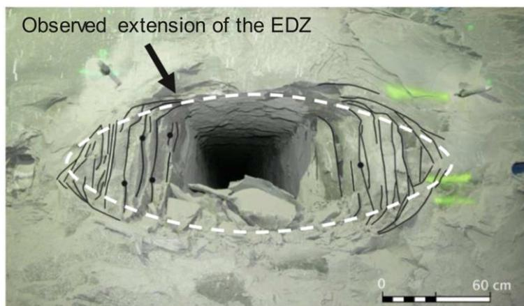
**Figure 8.** The observed fractures around the micro-tunnel in COx claystone induced by excavation. Reprinted from [5] with permission from Elsevier.
