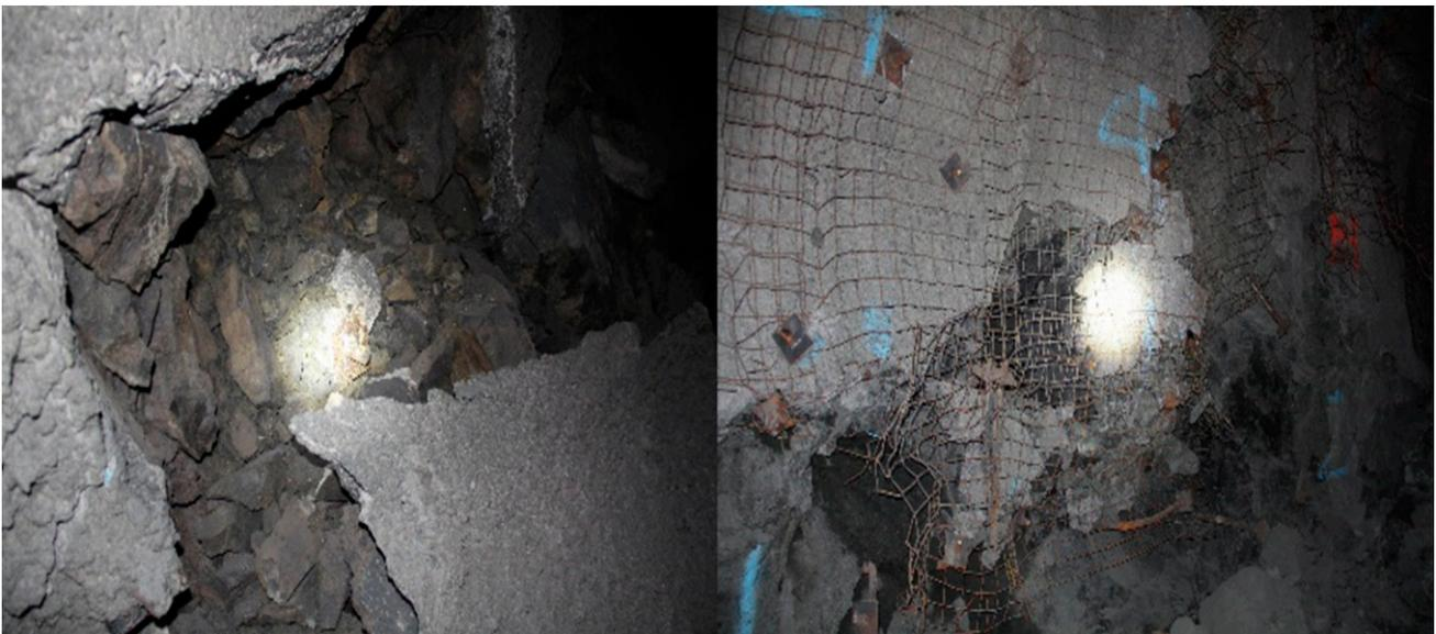
**Figure 10.** Failure cases near the stope access.
