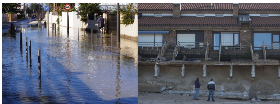
Figure 1. Buildings progressively damaged by extreme events. March 2014 storm (source: own collection).
