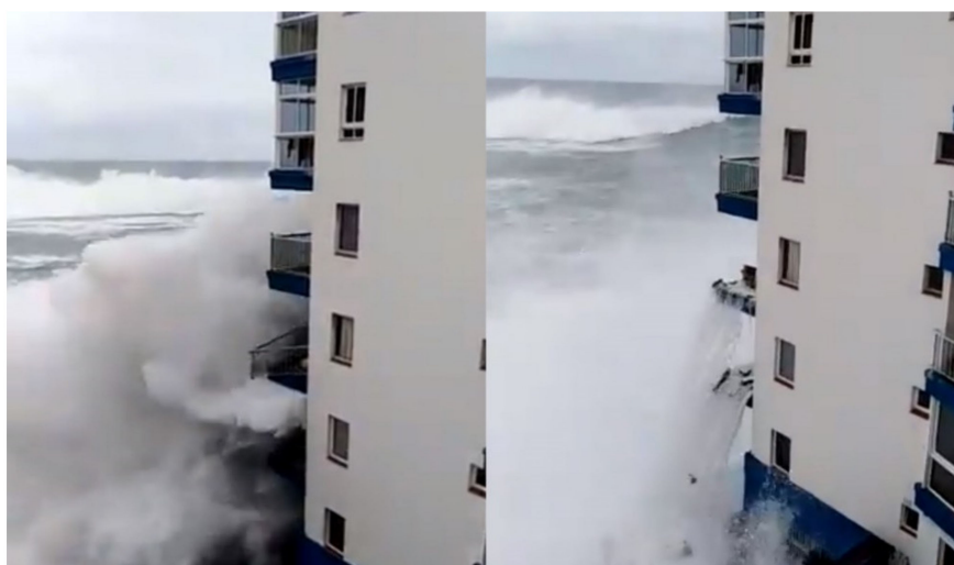
Figure 3. Action of the maritime climate on buildings right on the coast (Tacoronte, Spain, 2017). Source: own collection.
