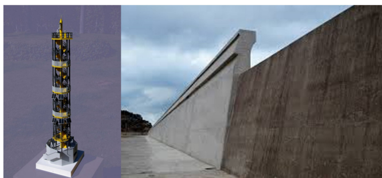
Figure 13. Composite materials lighthouse in Valencia (2015) and screed of the crown wall in Escombreras with FRP (2017) (source: own collection).
