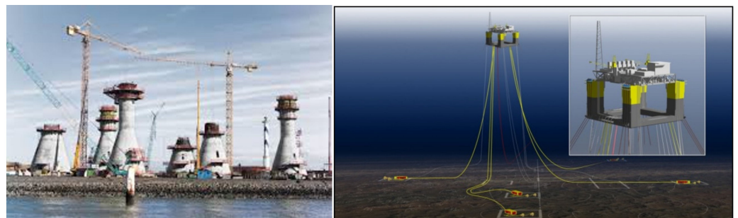
Figure 7. Difference between a GBS and a floating structure (Marinero 2018) [29].
