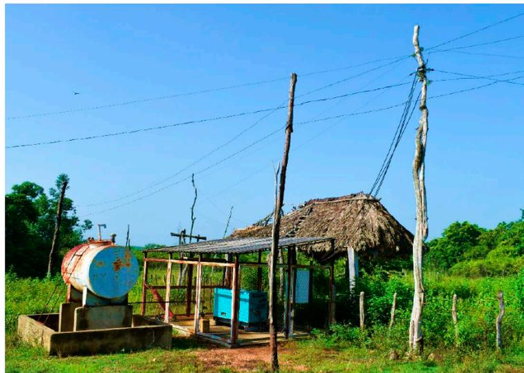
**Figure 3.** Generator set of 20 kVA (16 kW) and fuel storage tank in Yaguá.
