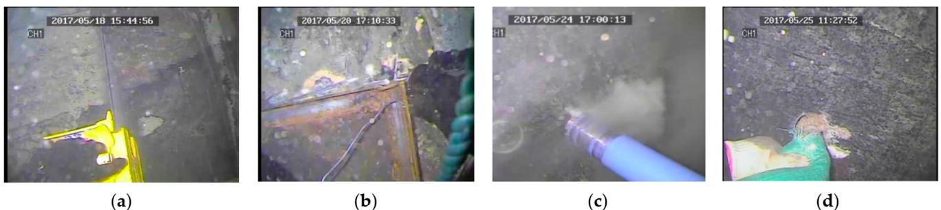
**Figure 6.** The construction process: (a) panel cutting; (b) die fixing; (c) construction panel drilling; (d) grouting.
