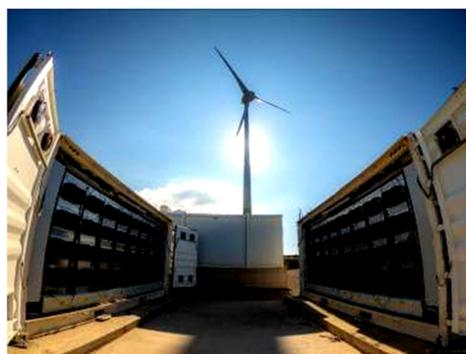
Figure 17. Photo of the Tilos HPS BESS, installed at the northwestern part of the island.
