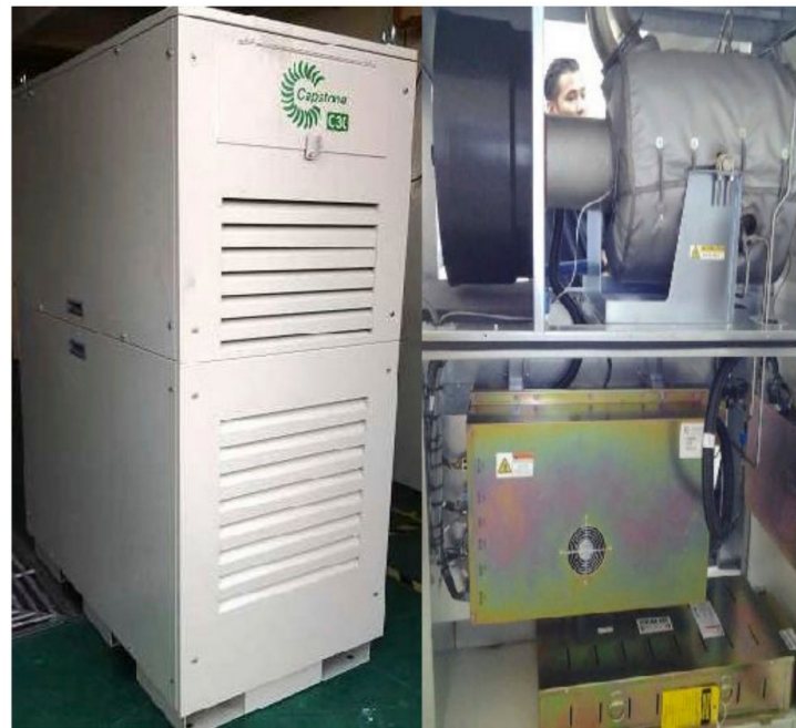
Figure 20. View of the Capstone 30 kW gas turbine [134].
