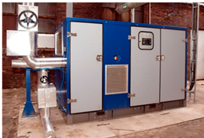
Figure 35. View of the screw expander made by Heliex Power installed at Zakłady Azotowe Kędzierzyn [164].
