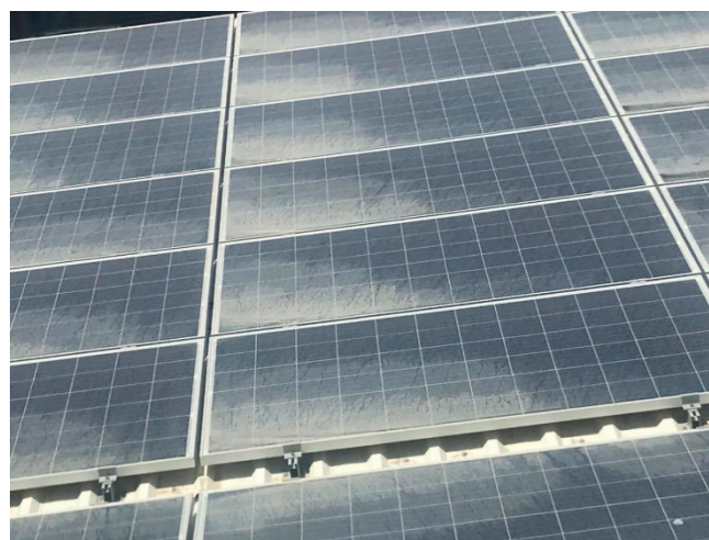
Figure 9. Photograph of partial section of the modules showing the high dust accumulation.
