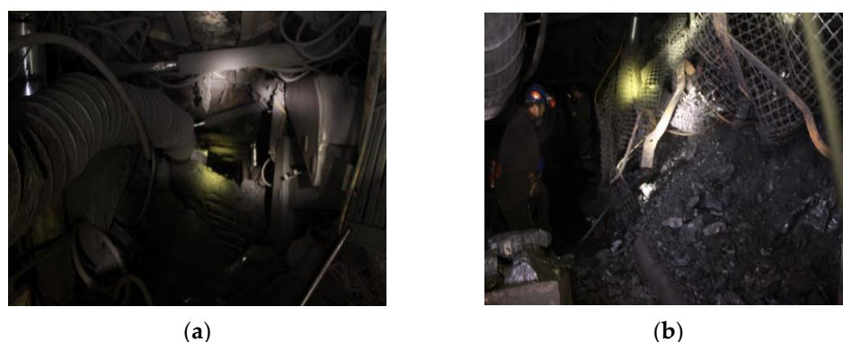
Figure 3. Damage situation at the No. 2 panel area. (a,b) support failure at roadway walls.
