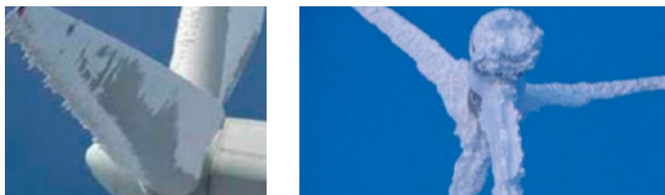
Figure 1. Examples of wind turbine icing.
