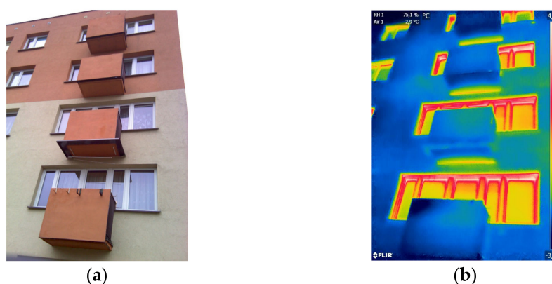
Figure 2. Fragment of the balcony facade of one of the analyzed large-panel residential buildings (OWT-67 system): (a) Photography; (b) Thermal image taken of the external wall surfaces of the building.
