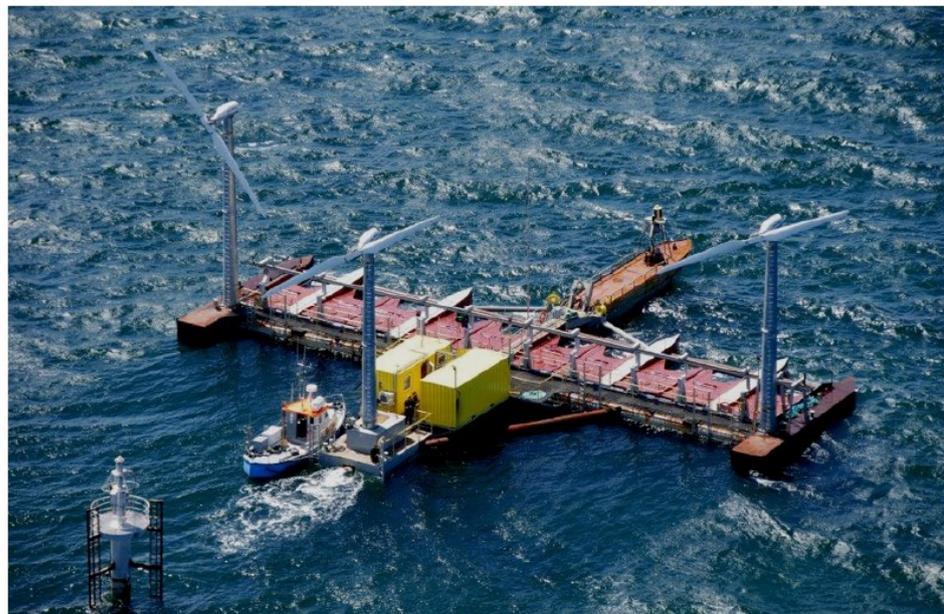
**Figure 7.** Poseidon hybrid wind–wave energy platform, developed by Floating Power Plant. Image taken from Ref. [44] “McTiernan, K.L.; Sharman, K.T. Review of Hybrid Offshore Wind and Wave Energy Systems. *J. Phys. Conf. Ser.* **2020**, *1452*, 012016.” Copyright 2020 Author(s), licensed under a Creative Commons Attribution (CC BY 3.0) license.
