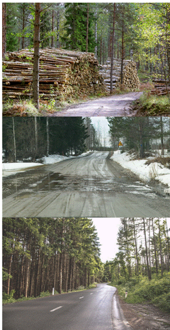
Figure S1. Three categories of road network in wood transportation: forest roads with speed \leq 30 km h -1 , rural gravel roads with speed >30 and < 60 km h -1 and 2nd class highway with speed \geq 60 km h -1 .
