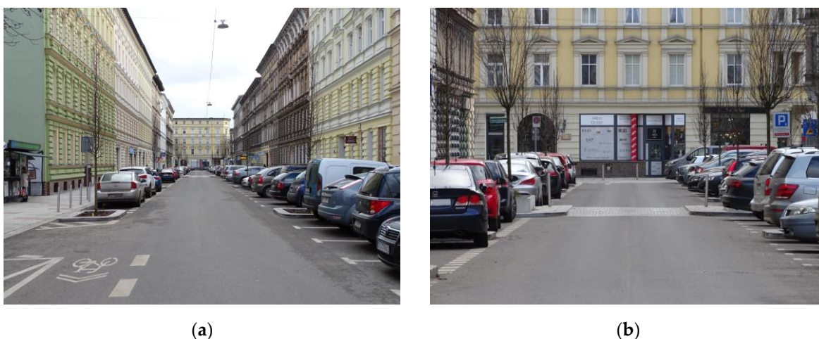
Figure 5. Test sections before and after chokers with raised pedestrian crossings in testing ground No. 1, No. 2 and No. 3: (a) test section before choker; (b) test section after choker. Source: own work of the author.
