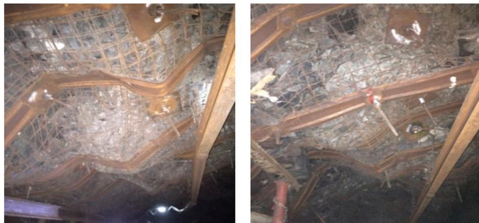
**Figure 3.** Deformation and failure characteristics of the roadway.
