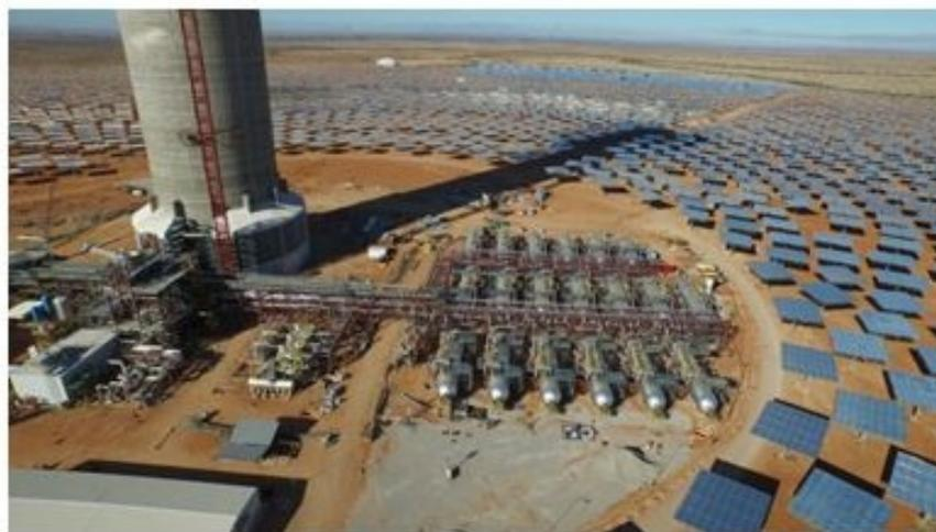
**Figure 3.** Steam accumulators of 50 MWe Khi Solar One plant (Source: Abengoa).
