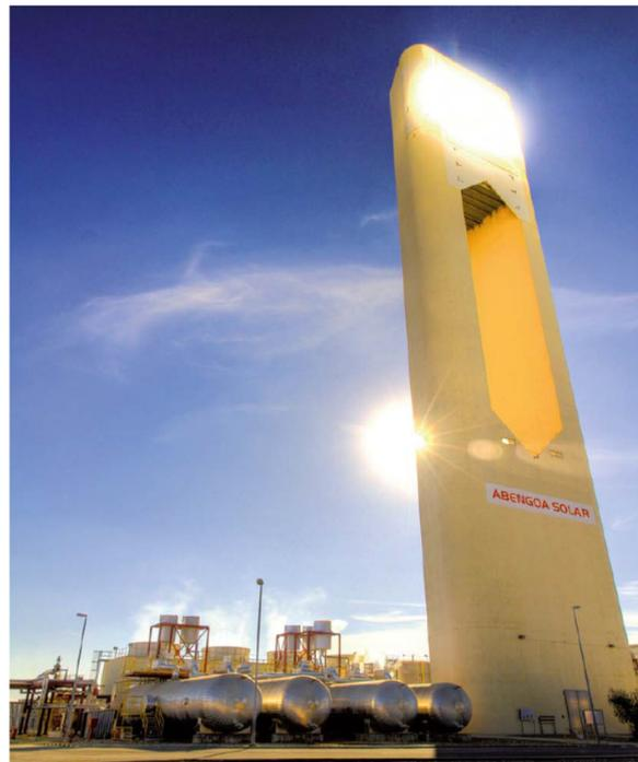
**Figure 2.** Steam accumulators of PS10 plant (Source: Abengoa).
