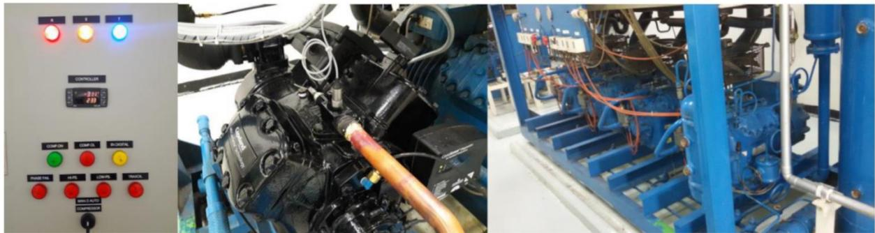
Figure 5. Digital compressor rack with digital compressor and digital controller No.1 (R404A).
