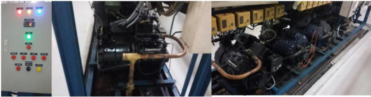
Figure 4. Digital compressor rack with digital compressor and digital controller No.1 (R22).
