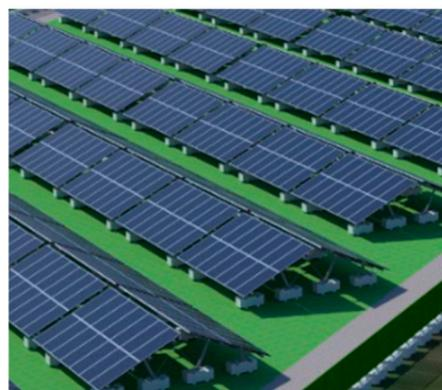
a) Gable Structure PV installation (Simulation)
