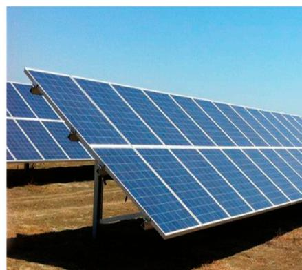
a) Fixed-tilt PV installation
