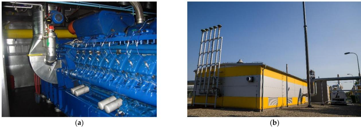
**Figure 2.** Gas engines (a) TBG 620V gas engine [38]; (b) in the Budryk mine.
