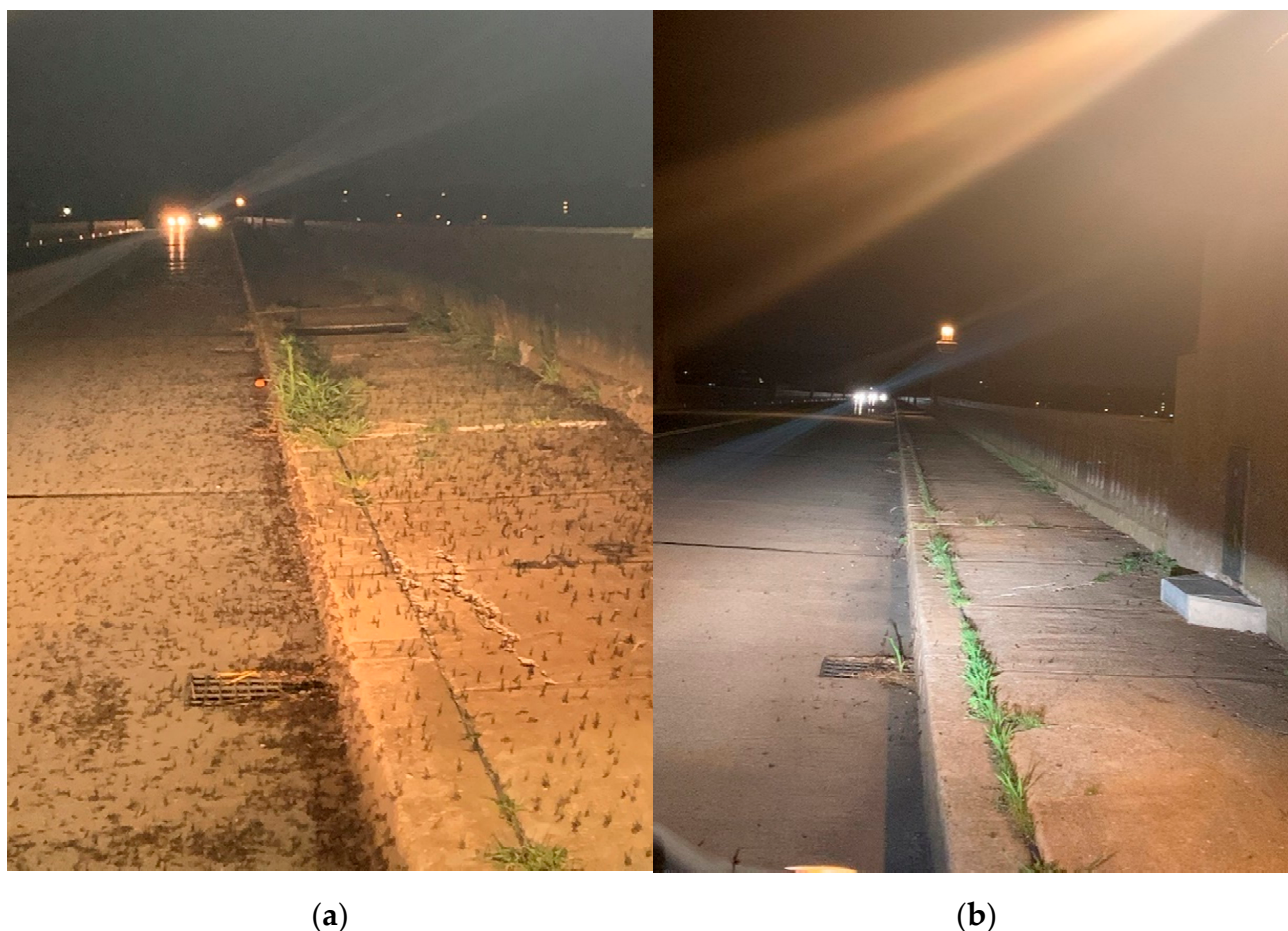
Figure 6. Photos of roadway and sidewalk near the base of the light fixtures on the piers of the Veterans Memorial Bridge: (a) at Span 12 (4800 K); (b) at Span 20 (2200 K) taken within minutes of each other during trial CW7. Visual observations suggested that more mayflies were attracted to the higher CCT light source (left image), despite no significant difference in statistical analysis between the trials. It should be noted that due to the car headlamps, the image on the right appears to be higher CCT, but the roadway luminaire in that image does indeed have the 2200 K light source.
