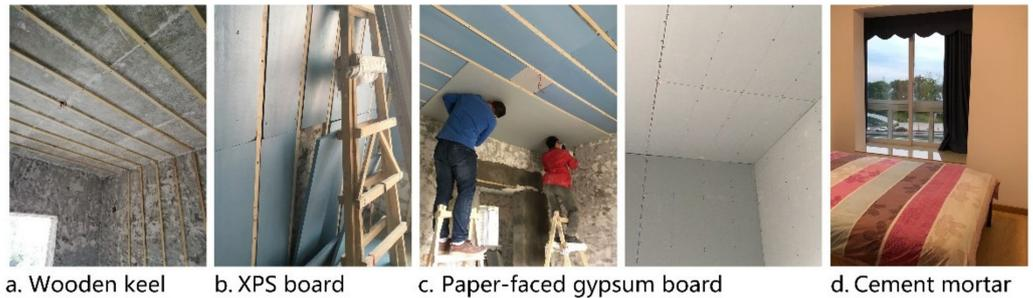
Figure 7. Overall view of the retrofit construction process.
