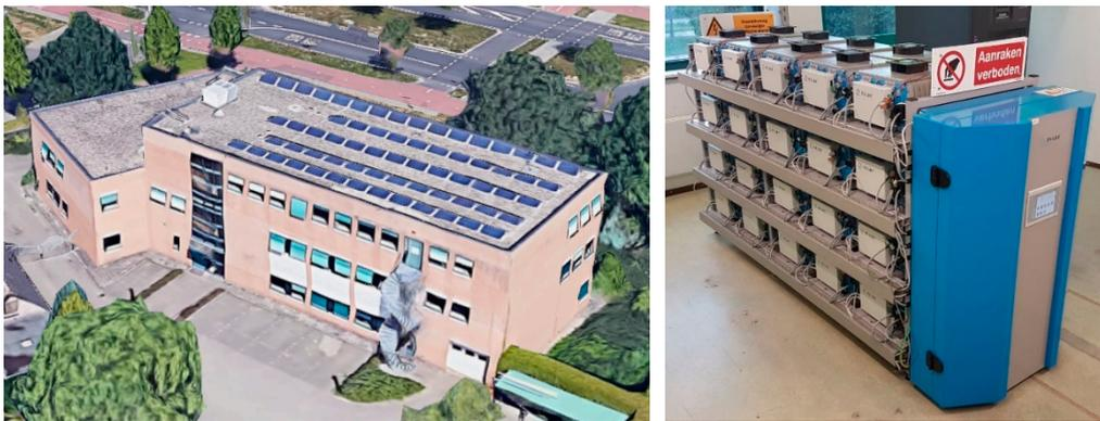
**Figure 1.** (Left) Impression of the building. (Right) A Battery Electric Storage System (BESS) installed inside the building.
