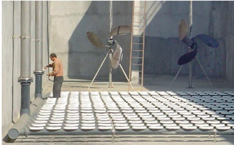
**Figure 1.** Fixed bottom aeration grid and agitators [5].
