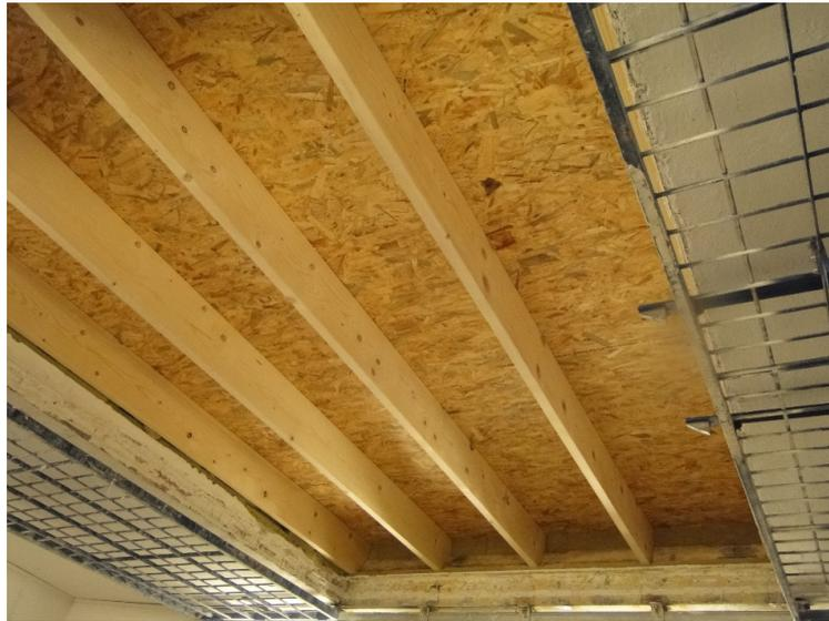
**Figure 4.** Basic construction of the wooden floor (model 1a) in a test facility.
