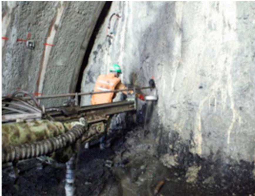
Figure 4. The hydraulic rotary percussion drill.
