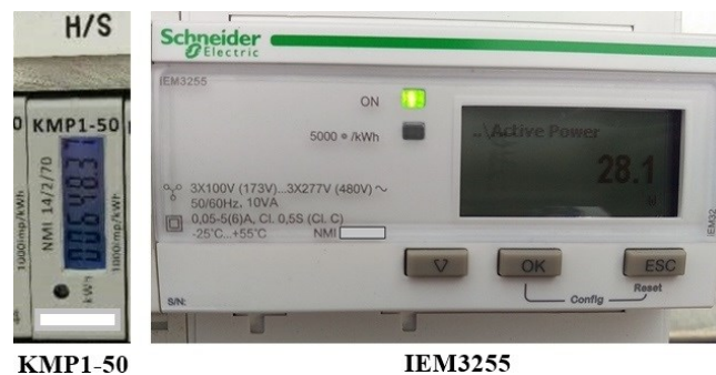
Figure 2. (a) Common property (CP) load connection to AC- and DC-coupled configurations. (b) Pulse meters used for measuring CP demand.
