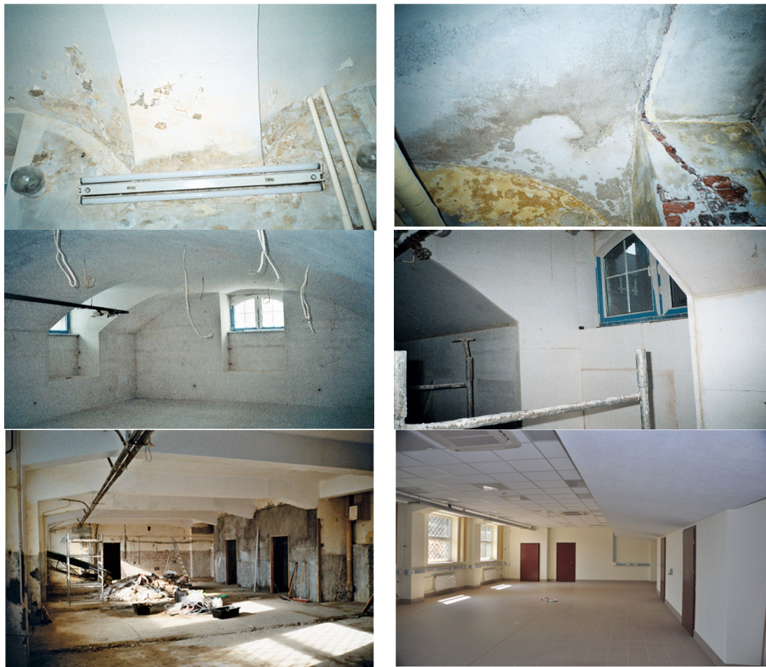
Figure 4. Photographs before, during and after the energy retrofitting process of selected cellar spaces.
