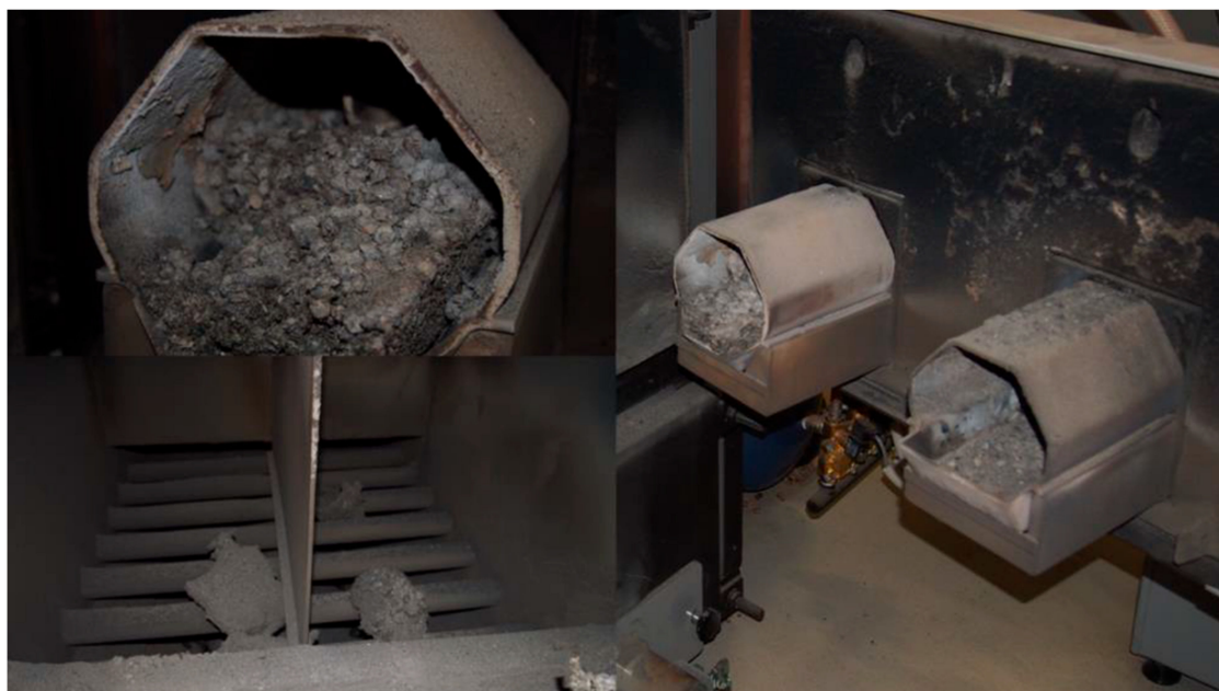
Figure 6. Effects of the incorrect combustion process—a view of the boiler combustion chamber and burners.
