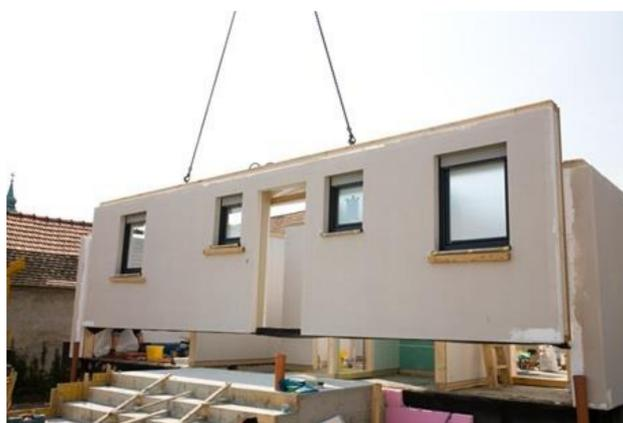
**Figure 1.** Prefabricated sandwich construction system [51].
