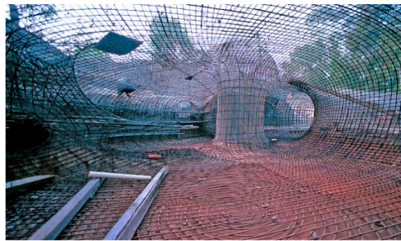
Figure 1. Internal structure based on anti-seismic rods.
