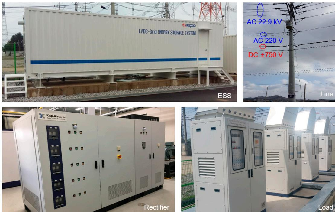
Figure 10. DC Components at the DC demonstration site.
