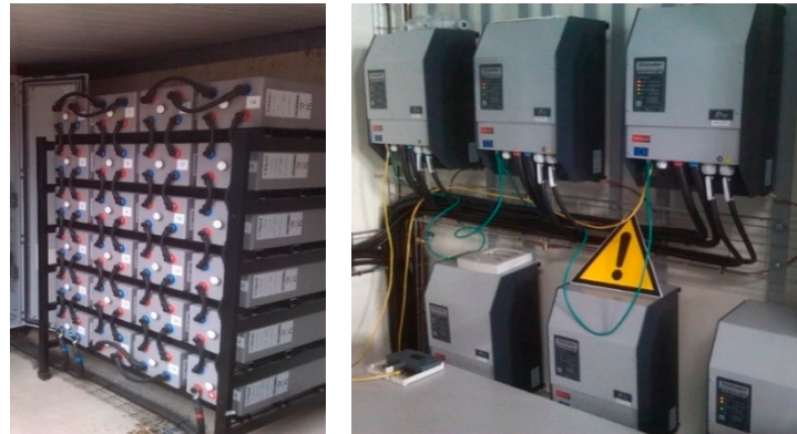
Figure 2. Energy Storage systems (ES): Batteries and inverters/chargers.
