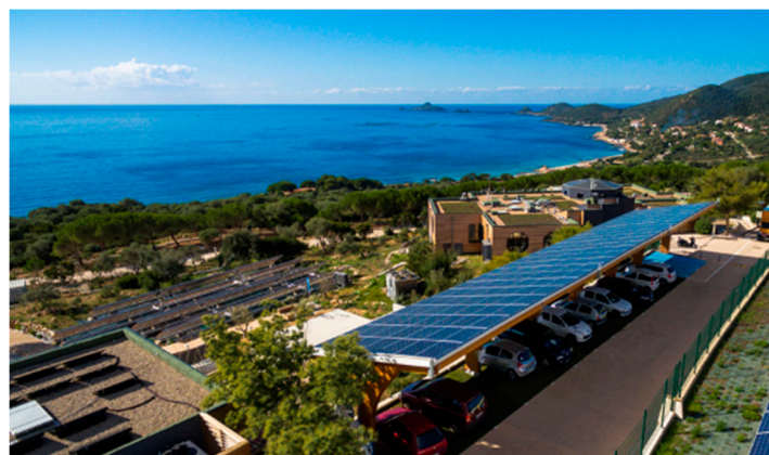
Figure 1. Distributed Generation systems (DG): Photovoltaic (PV) solar shade structure.
