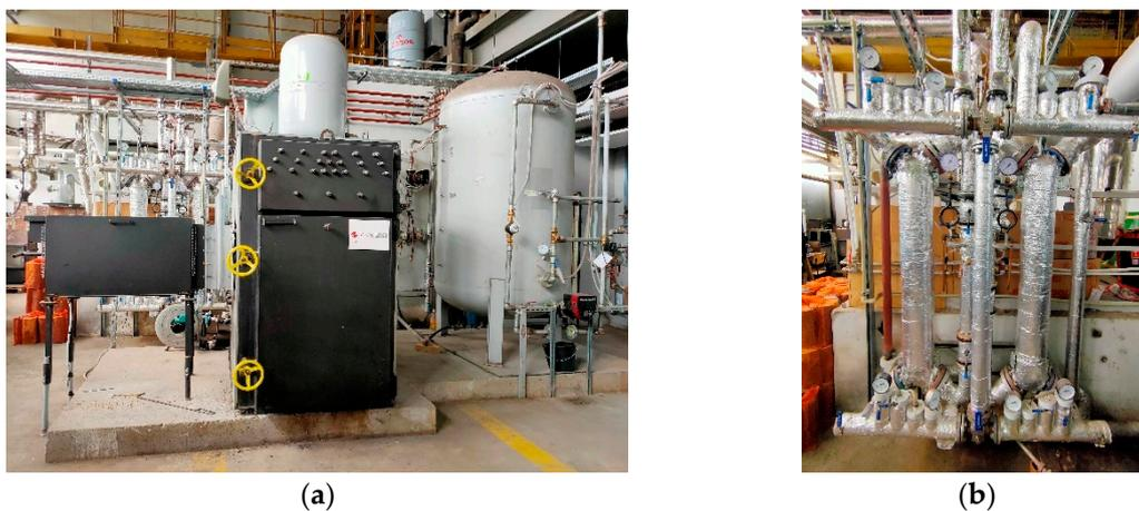
**Figure 4.** The view of (a) the boiler with a fuel feeder; (b) evaporator and superheater.
