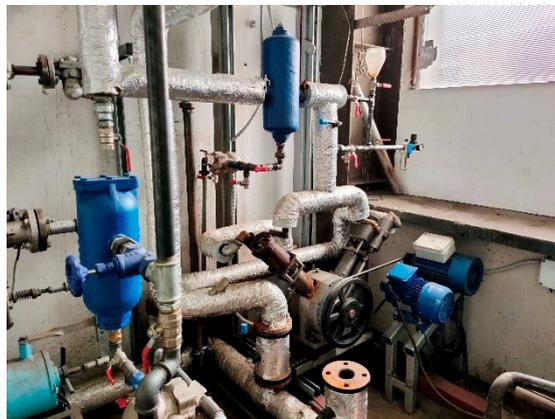
**Figure 3.** The steam engine and power generator used during the presented investigations.
