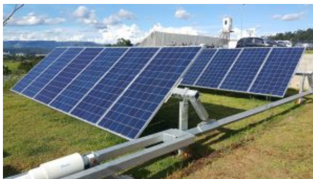
Figure 4. Horizontal single-axis tracker.
