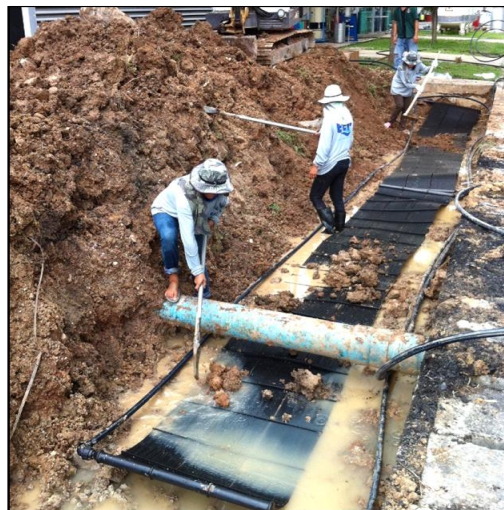
Figure 4. Carpet-type heat exchanger installation.
