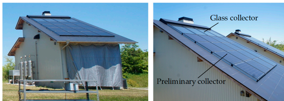
Figure 4. Target collector. Reproduced from [20], publisher: 2018.
