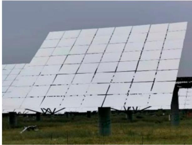
**Figure 4.** Surface shape of heliostat in the Yanqing CSP plant.
