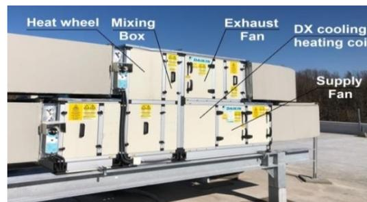
**Figure 1.** Photo from the investigated air handling units (AHU).
