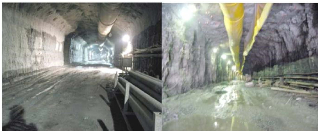
Figure 3. View of a mechanically driven heading (on the left) and a heading excavated using explosives (on the right) [1].
