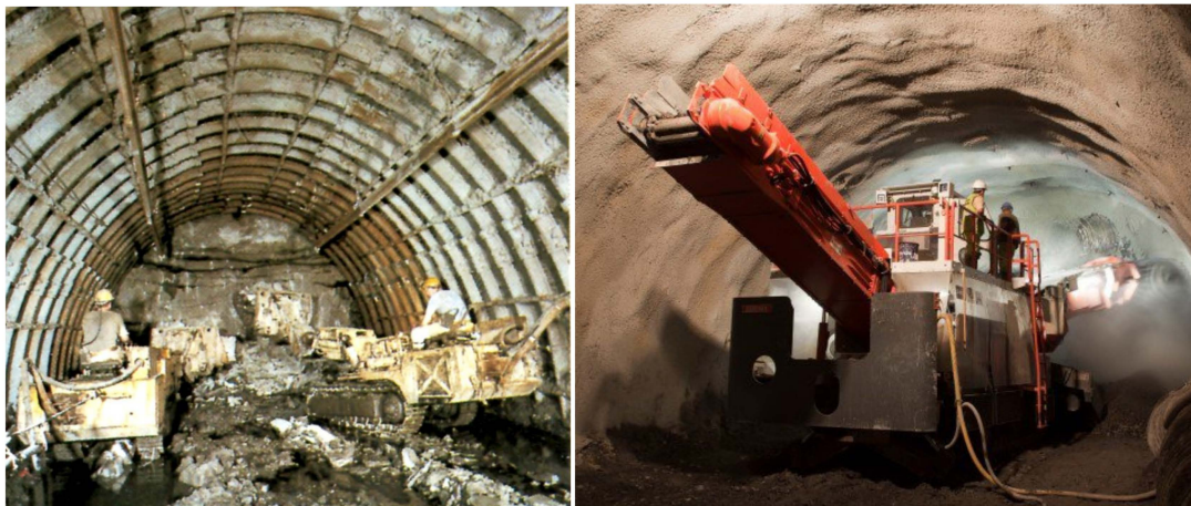
Figure 2. View of heading face driven using blasting material—left (drilling car and loader made by Deilmann Haniel), and mechanically—right (MT720 roadheader made by Sandvik) [4,7].
