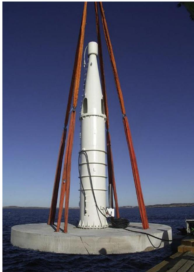
Figure 10. Deployment of the WEC developed by Uppsala university in the sea [6].
