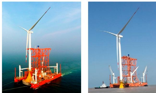
**Figure 2.** CBF with steel skirt of 3 MW in Xiangshui Wind Farm, Jiangsu Province, China.
