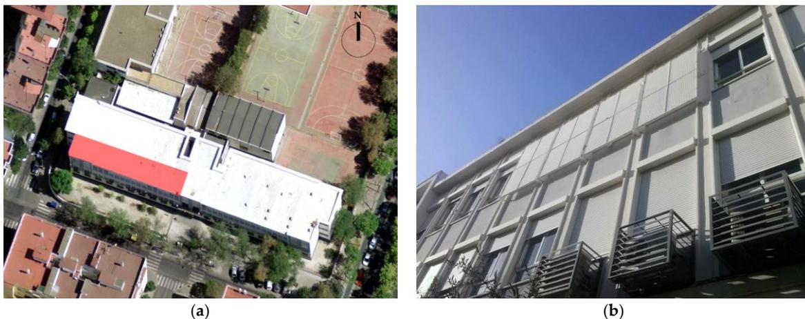
**Figure 1.** (a) Martínez Montañés Secondary School. The module of the classrooms monitored is shown in red. Base image: Google Earth Pro, 26 July 2017; (b) outdoor image of the rooms monitored: the four windows on the left, room without shading devices; the four windows on the right, and room with shading devices.
