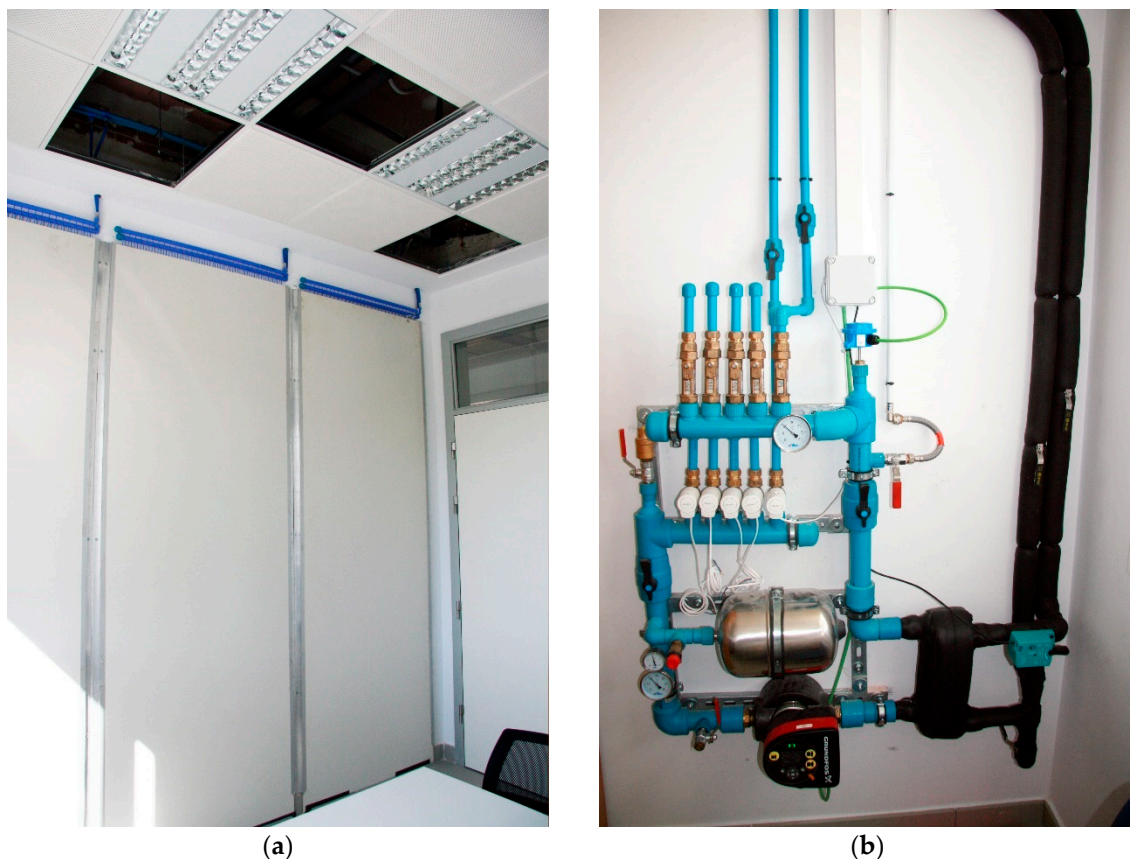
Figure 2. A thermal ceramic panel (TCP) in an office at Alicante University. (a) Distribution management substation. TCP panels in the standard office of the Multipurpose III building. University of Alicante; (b) Substation for management and control of distribution circuits.
