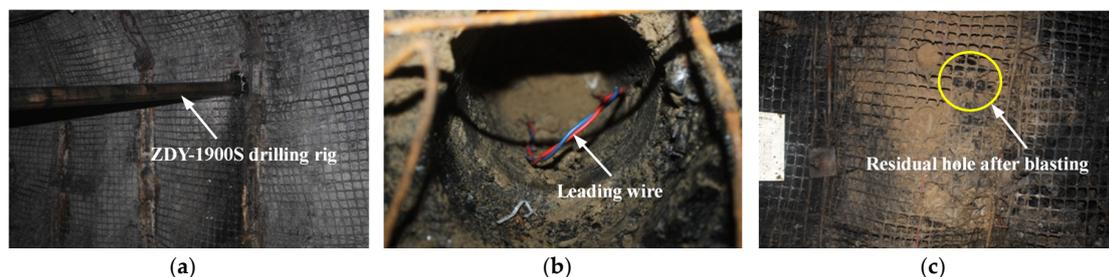
**Figure 14.** Practical application of DHB at the 4301 working face. (a) Blasting hole drilling; (b) Blasting hole charging; (c) Residual hole after blasting.
