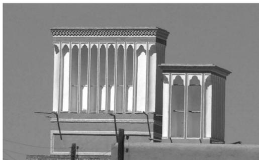
**Figure 1.** Two four-sided wind towers in Yazd, Iran [3].
