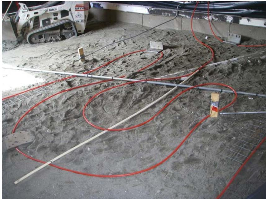
Figure 7. Cross-linked polyethylene (PEX) heat loop installation in progress.
