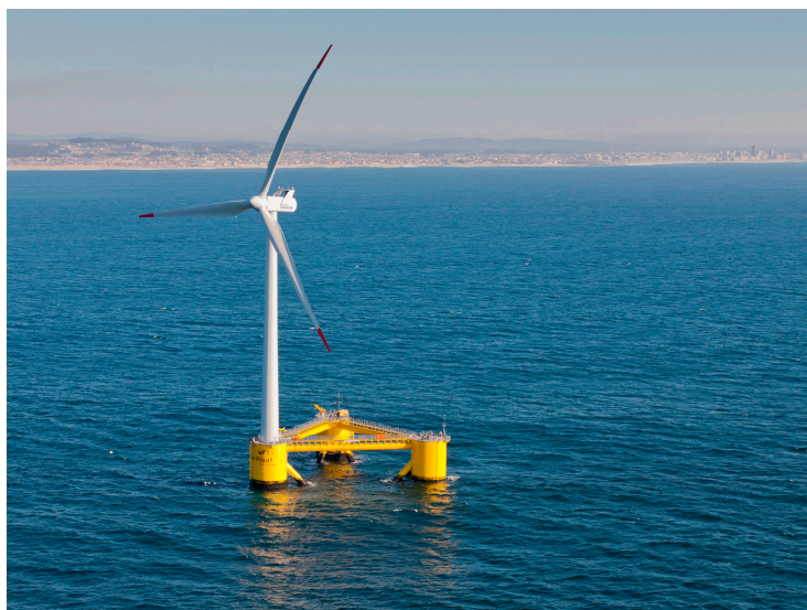
Figure 1. WindFloat: a semisubmersible floating 2 MW offshore wind turbine installation offshore Aguçadoura, Portugal. (Source: A semi-submersible type floating offshore wind turbine foundation called the WindFloat operating at rated capacity (2 MW) approximately 5 km offshore of Agucadoura, Portugal by Untrakdrover, retrieved from https://en.wikipedia.org/wiki/File:Agucadoura_WindFloat_Prototype.jpg . Used under Creative Commons Attribution-Share Alike 3.0 Unported license).
