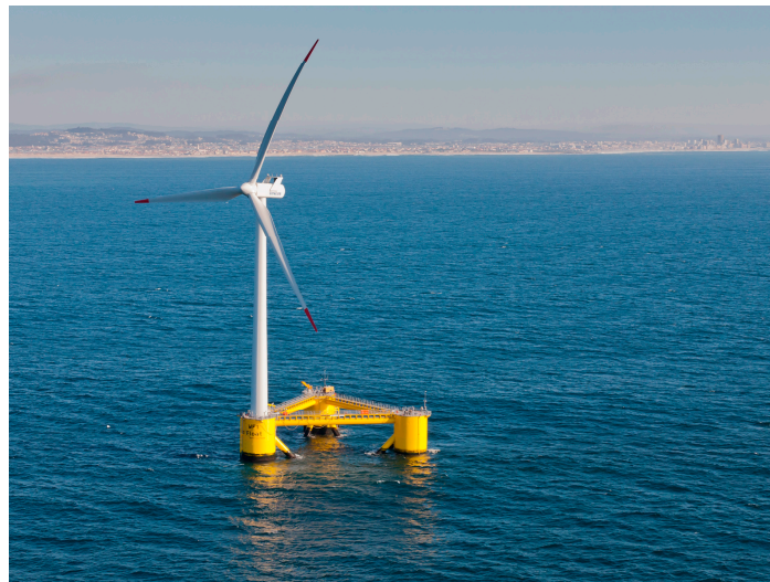
Figure 1. WindFloat: a semisubmersible floating 2 MW offshore wind turbine installation offshore Agucadoura, Portugal. (Source: A semi-submersible type floating offshore wind turbine foundation called the WindFloat operating at rated capacity (2 MW) approximately 5 km offshore of Agucadoura, Portugal by Untrakdrover, retrieved from https://en.wikipedia.org/wiki/File:Agucadoura_WindFloat_Prototype.jpg . Used under Creative Commons Attribution-Share Alike 3.0 Unported license).
