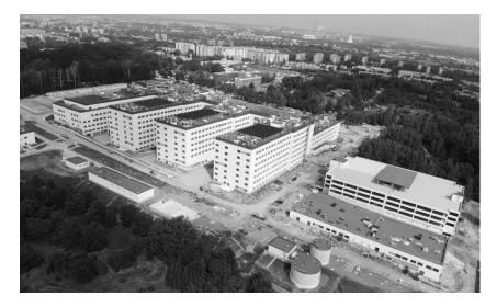
**Figure 5.** Comb layout (finger-plan) of the University Hospital in Prokocim, Kraków. Source: www.su.krakow.pl (accessed on 1 September 2021).
