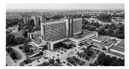
**Figure 7.** Tower-on-a-podium layout: Rydygiera Hospital in Krakow. Source: lovekrakow.pl (accessed on 1 September 2021).
