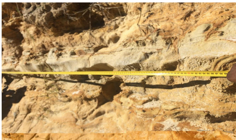
Figure 5. The side view surface of the dam showing cracks and fissures.
